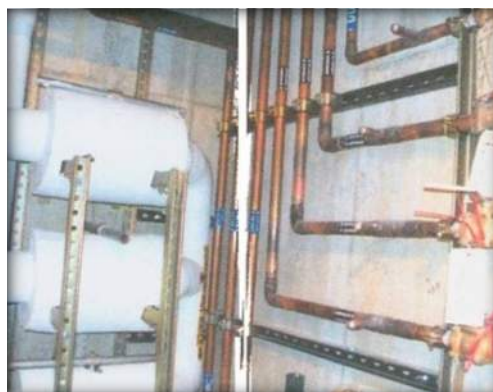
Nitrogen and nitrous oxide gas pipe.
