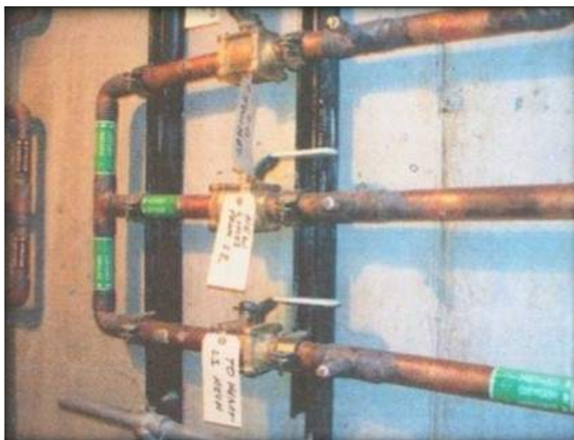
Piping loop valve assembly at a coronary heart hospital.
